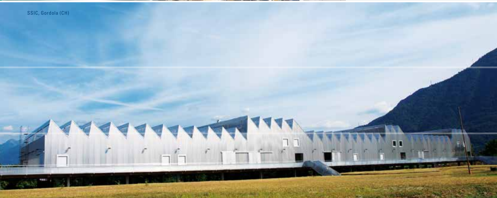
Brütsch Rüegger Toolcenter, Urdorf (CH)
